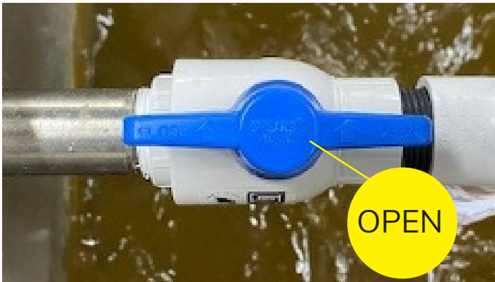
Sump Drain Valve (Open)
